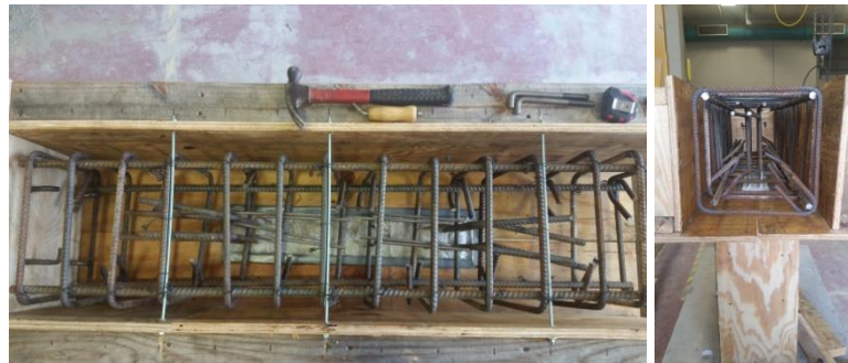
Figure 30 - Top block reinforcement
