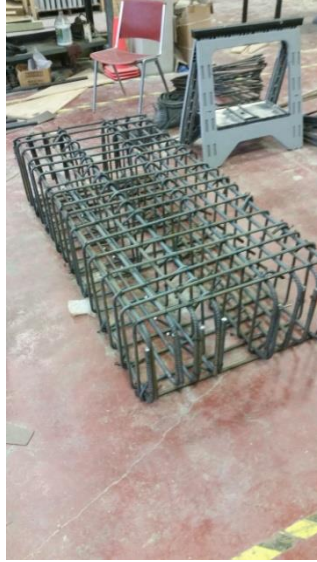
Figure 23 - Foundation reinforcement cage
