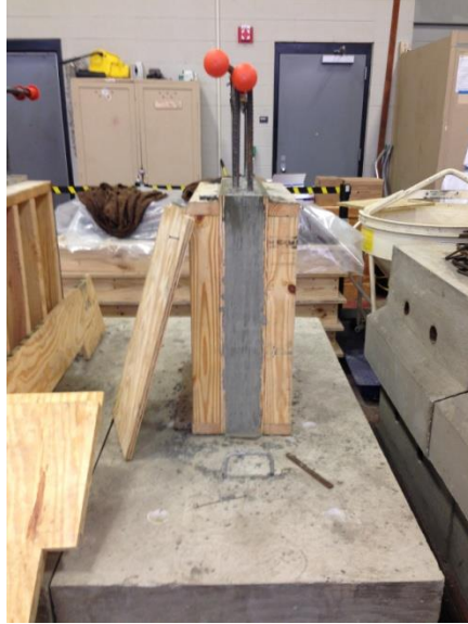
Figure 29 - Cast wall within formwork
