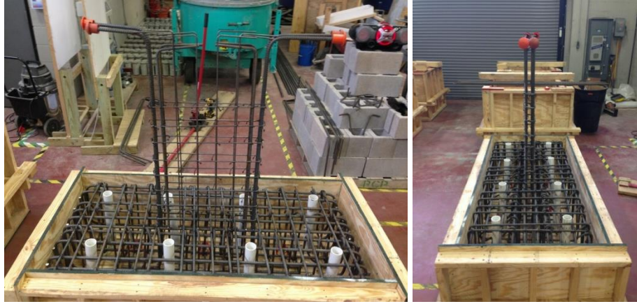
Figure 25 - PVC locations in foundations
