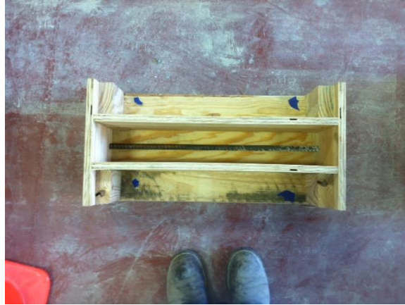
Figure 14 - Wooden formwork and rebar
