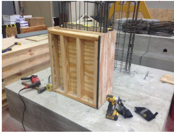
Figure 28 - Wall formwork
